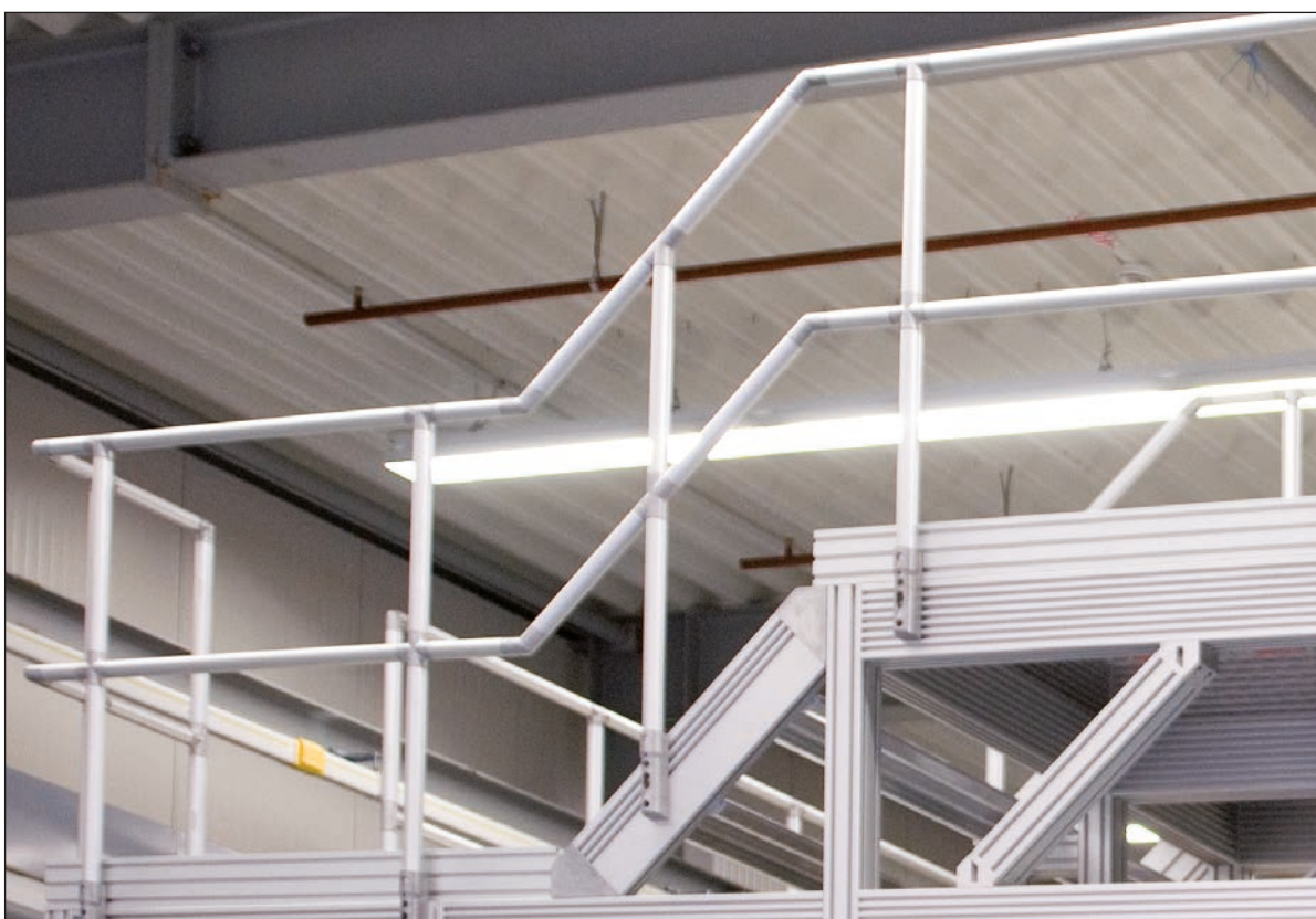
Staircase between two operating platforms.
