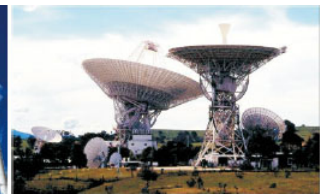
Radar Monitoring System
